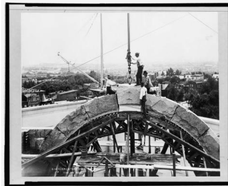
Men placing the keystone in the center of a stone arch.
