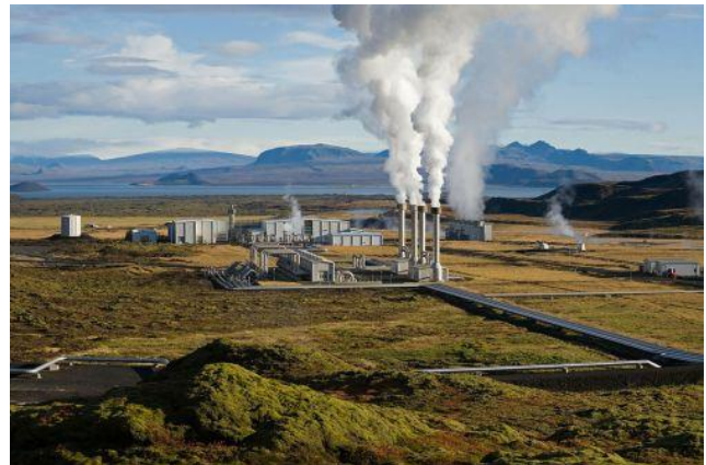
Geothermal power plant
