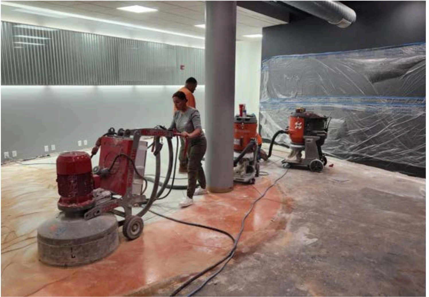
Contractor SI Legacy is really making progress, 5/1/24.
