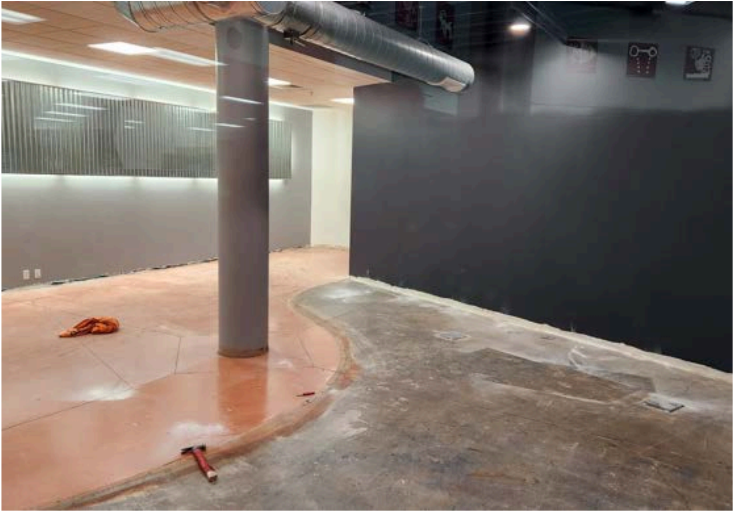
Reflooring work begins 5/1/24 with carpet removal.
