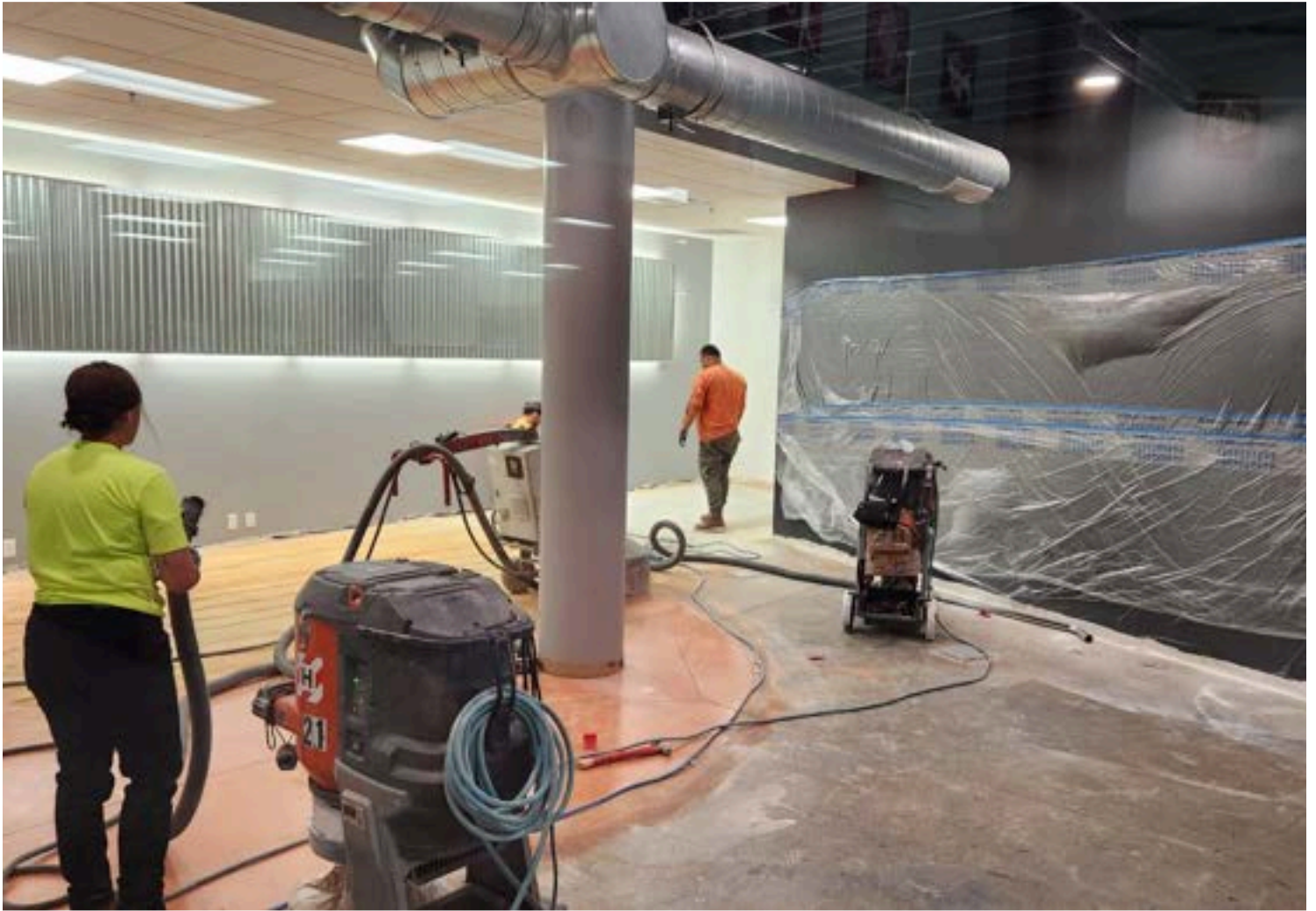
Next the painted surface is removed, 5/1/24.
