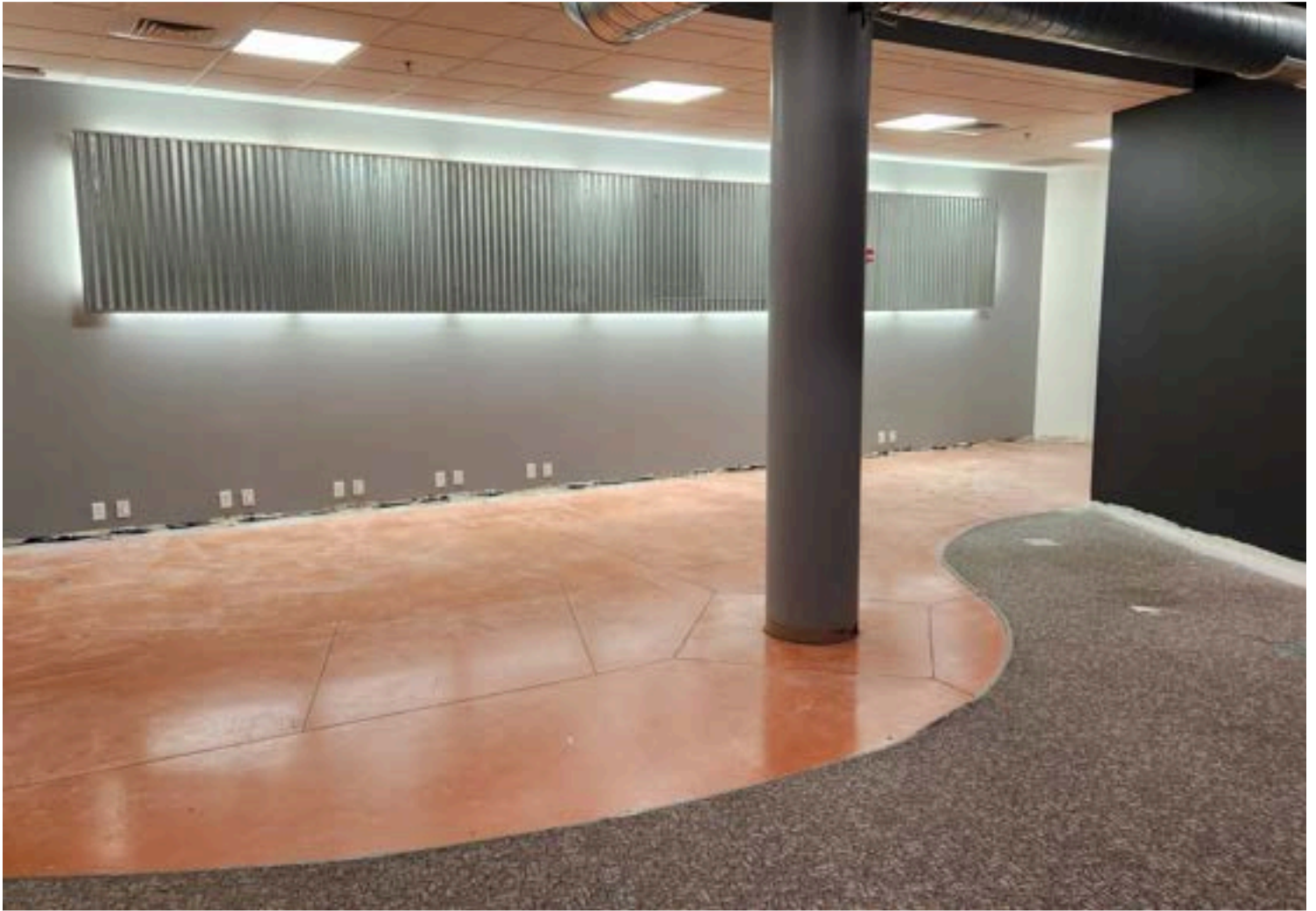
Our teen area is all cleared and ready for reflooring!
